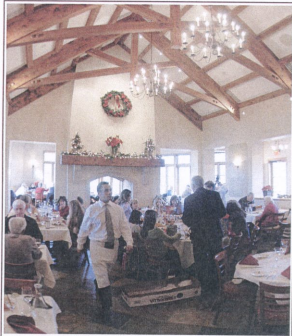
Reclaimed Douglas Fir trusses form an eye-catching arch over the LA Provence dining room in West Roseville
